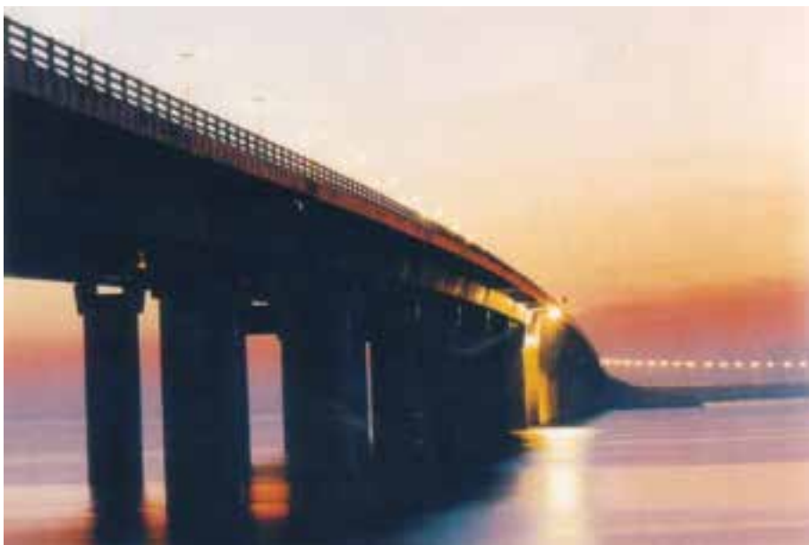
The King Fahd Bridge which connects Saudi Arabia to Bahrain.
